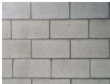
Cement Block Wall
